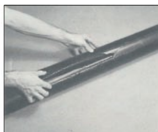
Encapsulate cable with FRE ® Split Conduit*
